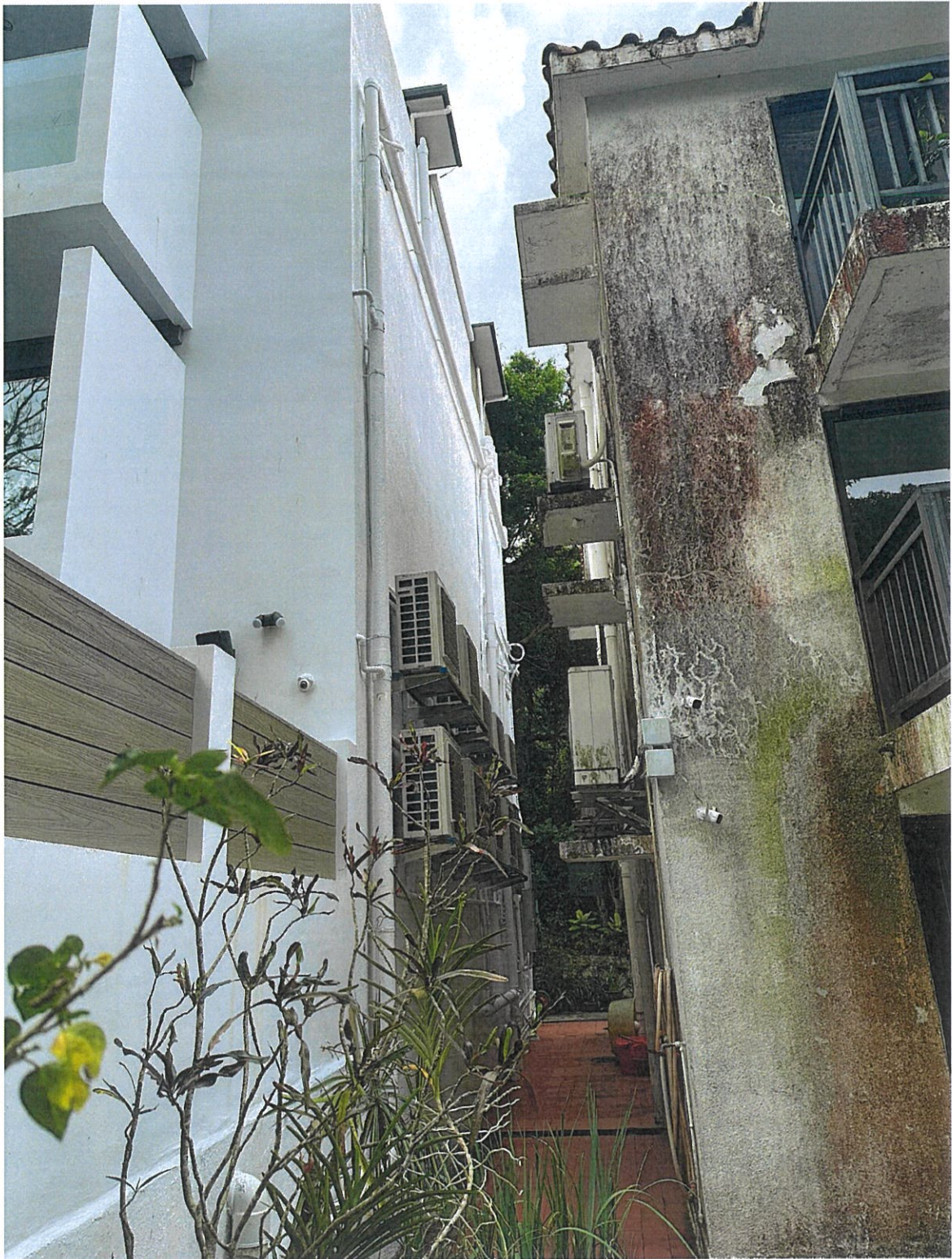
Picture 23 above shows a similar view after the renovation
