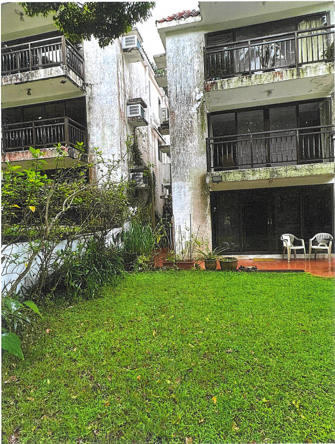
Picture 21 shows the 2 houses prior to renovation
