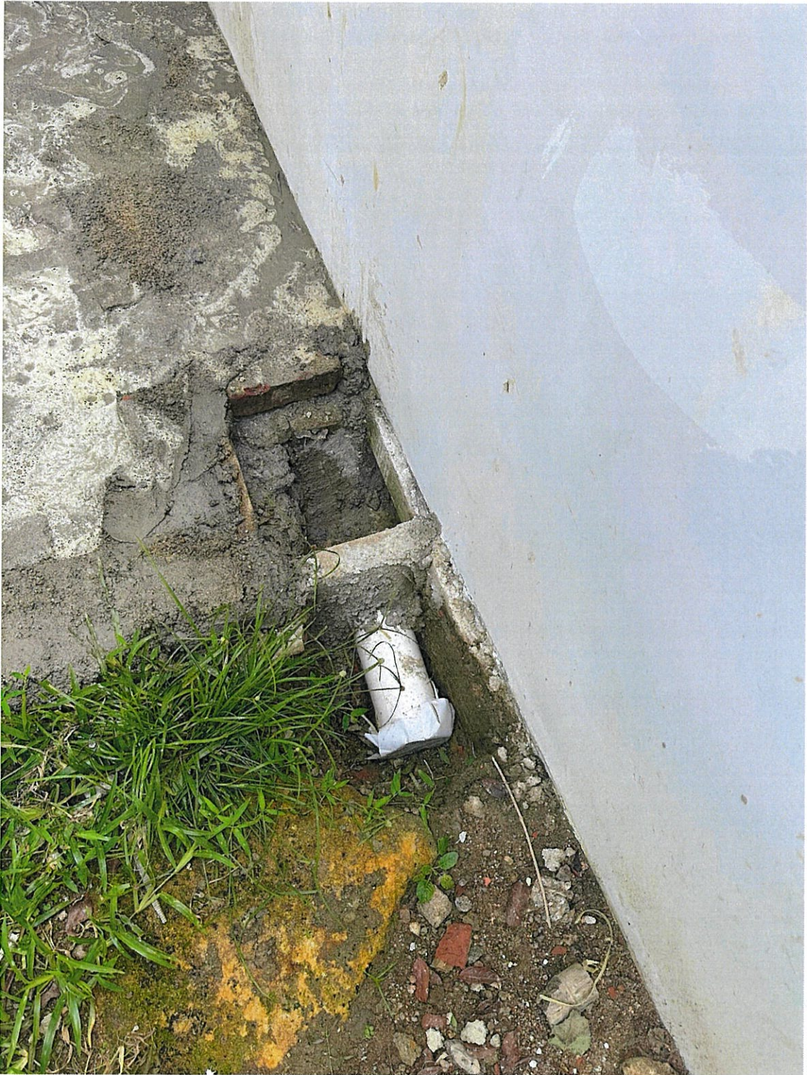
Picture 8 shows an additional drainage pipe, connecting to the existing drainage.
